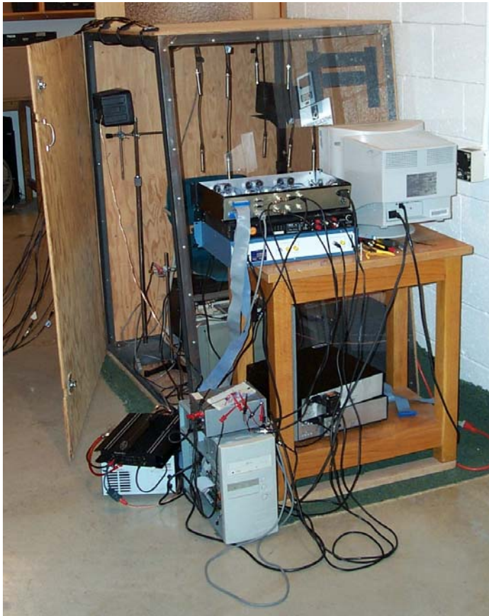
Figure 2. Mock cab and noise control system electronics.
