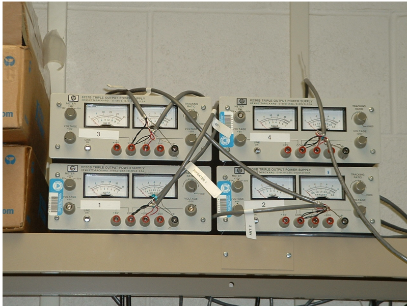
Figure 2.8: The four power supply boxes sit above Computer A. Each is labeled 1 through 4 respectively to its antenna.
