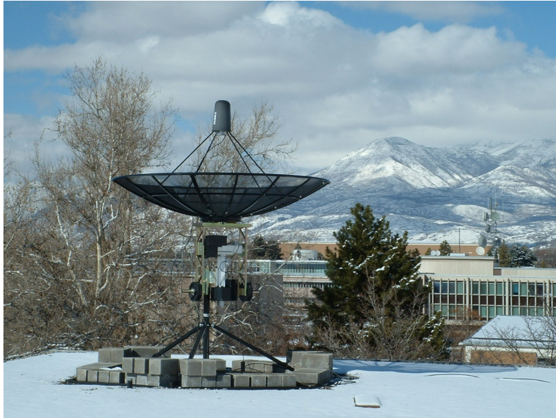
Figure 3.1: Antenna 1 (Eve) sits on the north-west corner of the Clyde Building.
