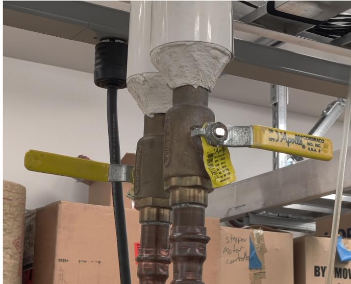
**Figure A.4** The water line valve handles. Twist them so they both point up to open the valves.
