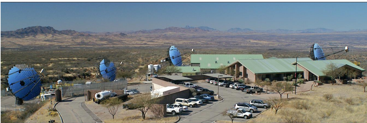
Figure 3: VERITAS is an array of four Cherenkov telescopes located in Southern Arizona. Each telescope has a dish of mirrors measuring 12 m and a camera composed of 499 photomultiplier tubes.
