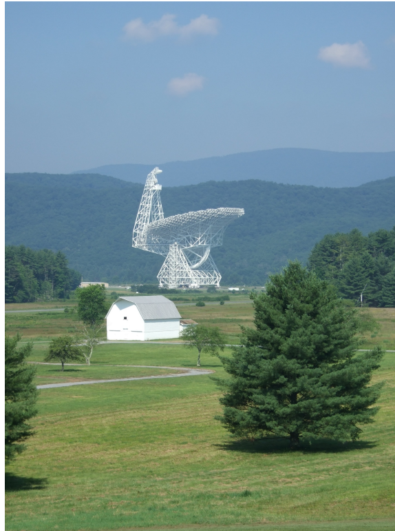
Figure 2.7 This is the Robert C. Byrd Green Bank Telescope (GBT). With its enormous 100-meter diameter dish, the GBT is the largest fully steerable telescope in the world. Photograph provided by the author.
