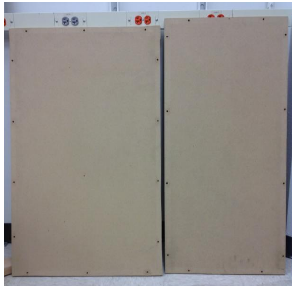
Figure 3.2 – Aperture panels used to close a side aperture (left) and front aperture (right).
