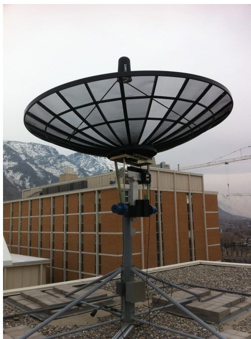
Figure 1.2 The 4 meter antenna on top of the ESC. This is at our AOC.
