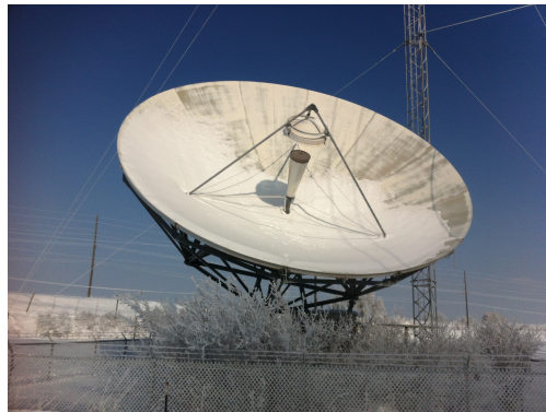
Figure 1.5 The 10 meter antenna in Spanish Fork, UT. This is currently unidirectional, so we will be undertaking the project to make it pointable.
