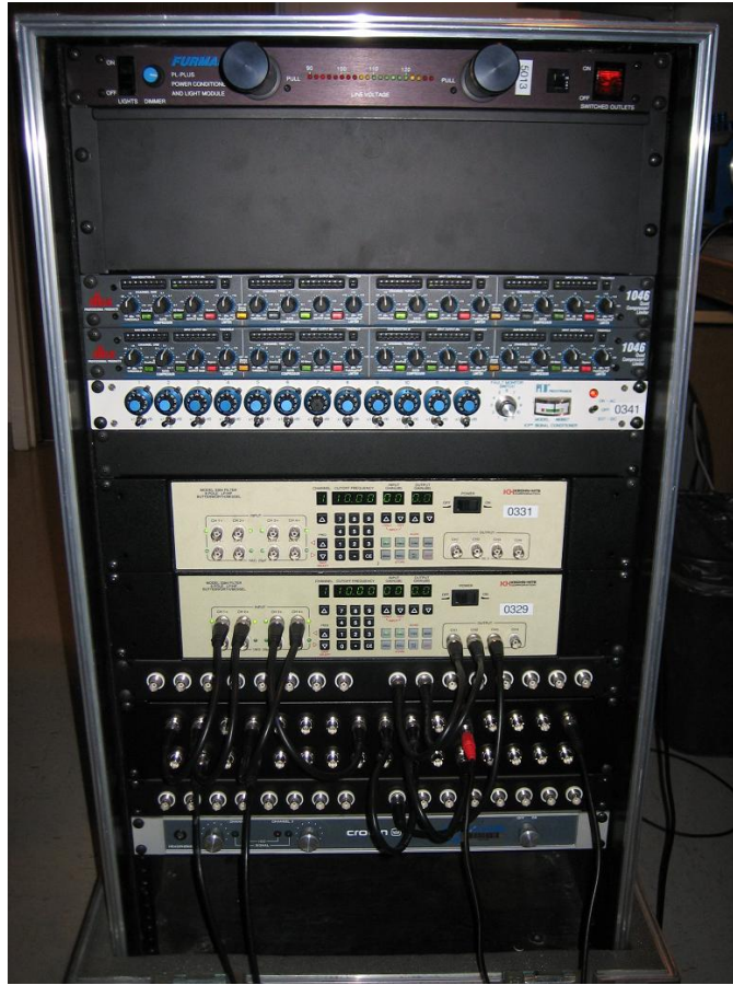
Figure 3.3 The Rack Setup
