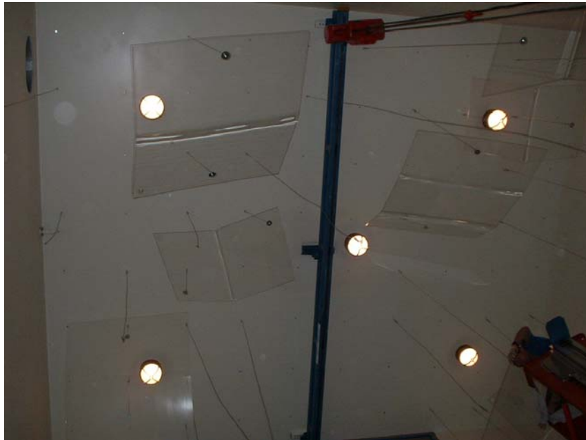
FIG. 2.1. Ceiling view of suspended diffuser panels in large chamber.
